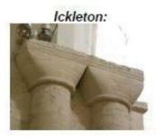
During the 13th-century damage was caused, still visible today, when mouldings were cut away for the installation of altars (SECH, 1994).
